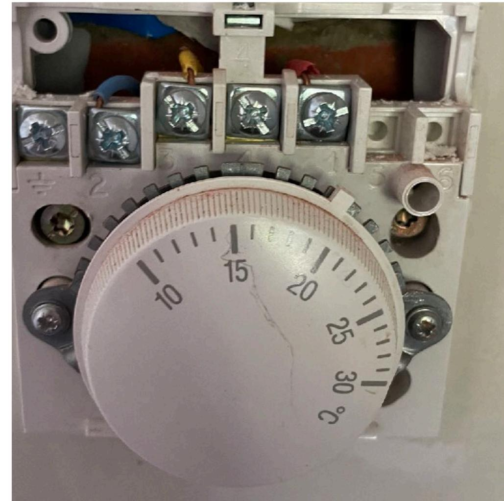
5. Disconnect call, live & neutral wires on room stat and remove stat
