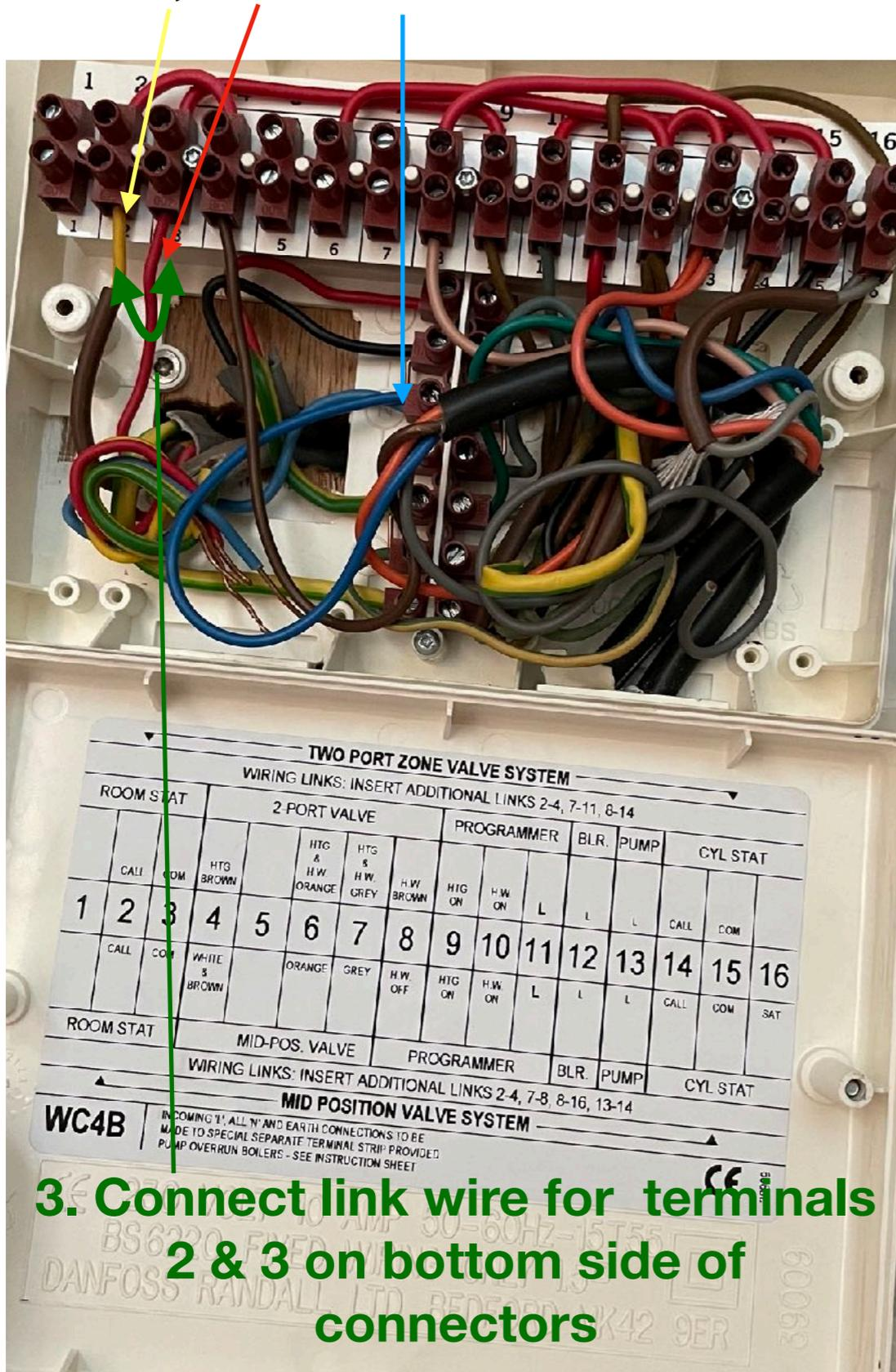
3. Connect link wire for terminals 2 & 3 on bottom side of connectors
